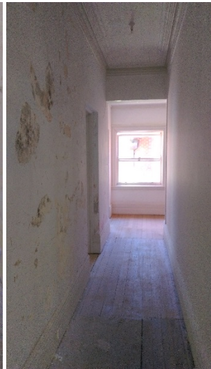
Typical Wall paint damage
