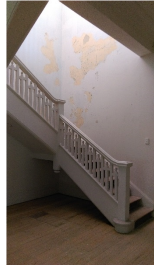
Typical Wall paint damage
